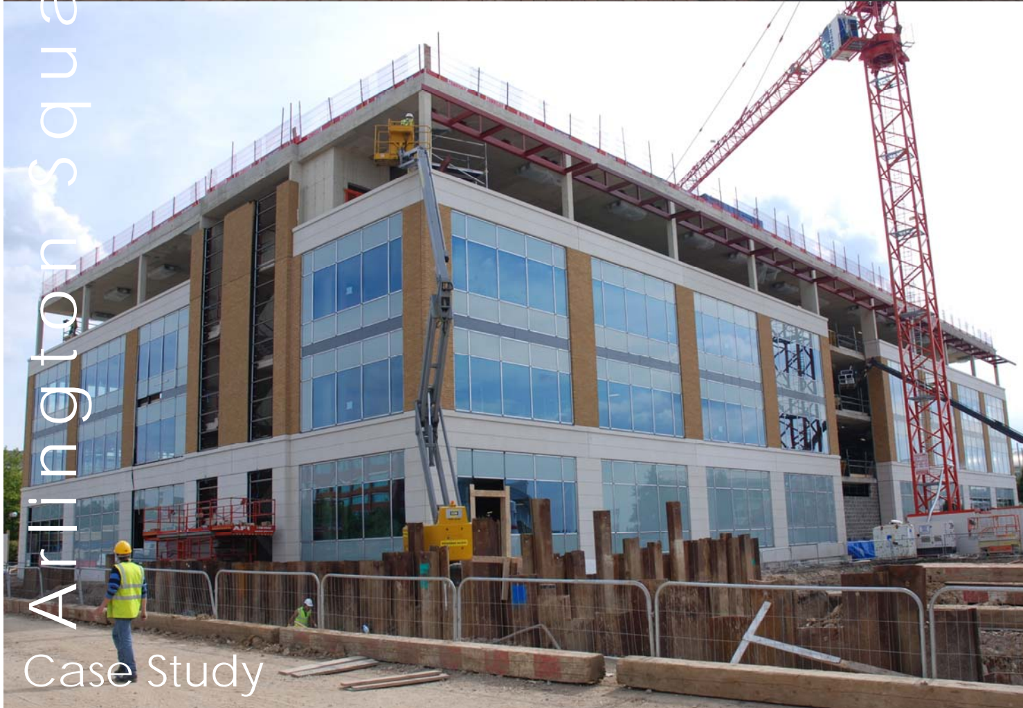
Brackets are fixed to cast in Halfen channels free issued to the main contractor by ourselves. Once panels have been checked for line and level, all bolts are locked off and sprayed as part of a QA procedure.
