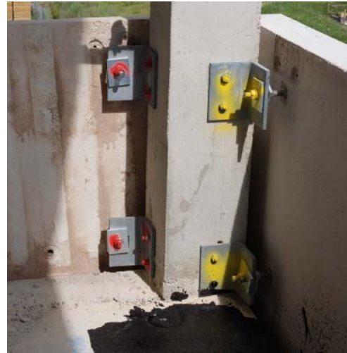
Brackets are fixed to cast in Halfen channels free issued to the main contractor by ourselves. Once panels have been checked for line and level, all bolts are locked off and sprayed as part of a QA procedure.
