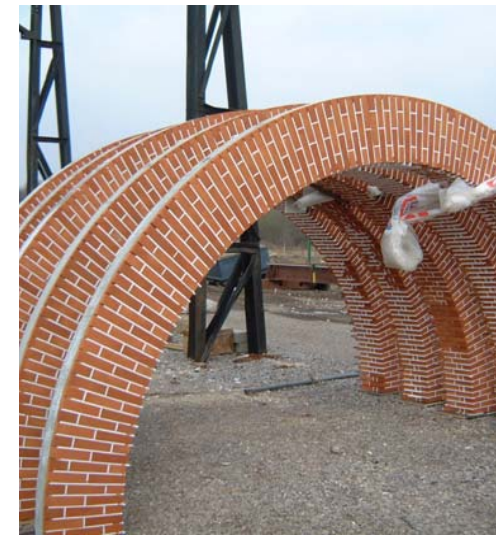
Arches manufactured and stored on the yard awaiting pointing and delivery.
