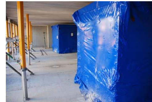
Bathroom pods are installed prior to precast floors being erected.
