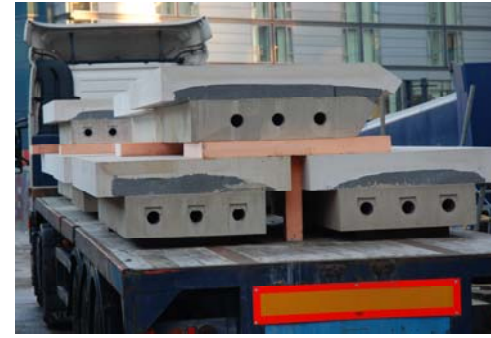
Structural cladding elements supplied as insulated sandwich panel.
