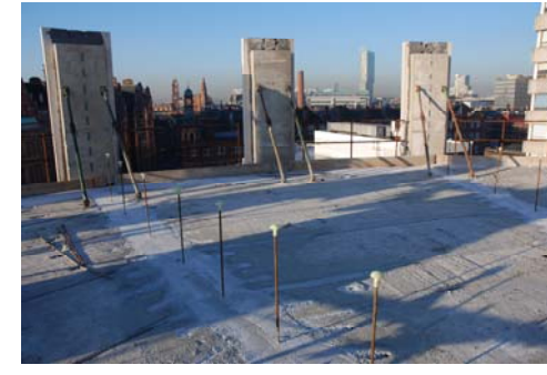
External mullions erected on push pull props.
