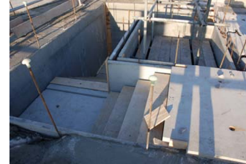
Supply of structural stair units complete with plywood protection.
