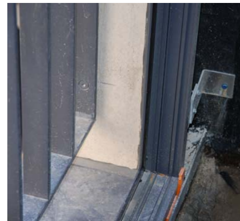
Glazing system fixed from within the building included mastic seal application
