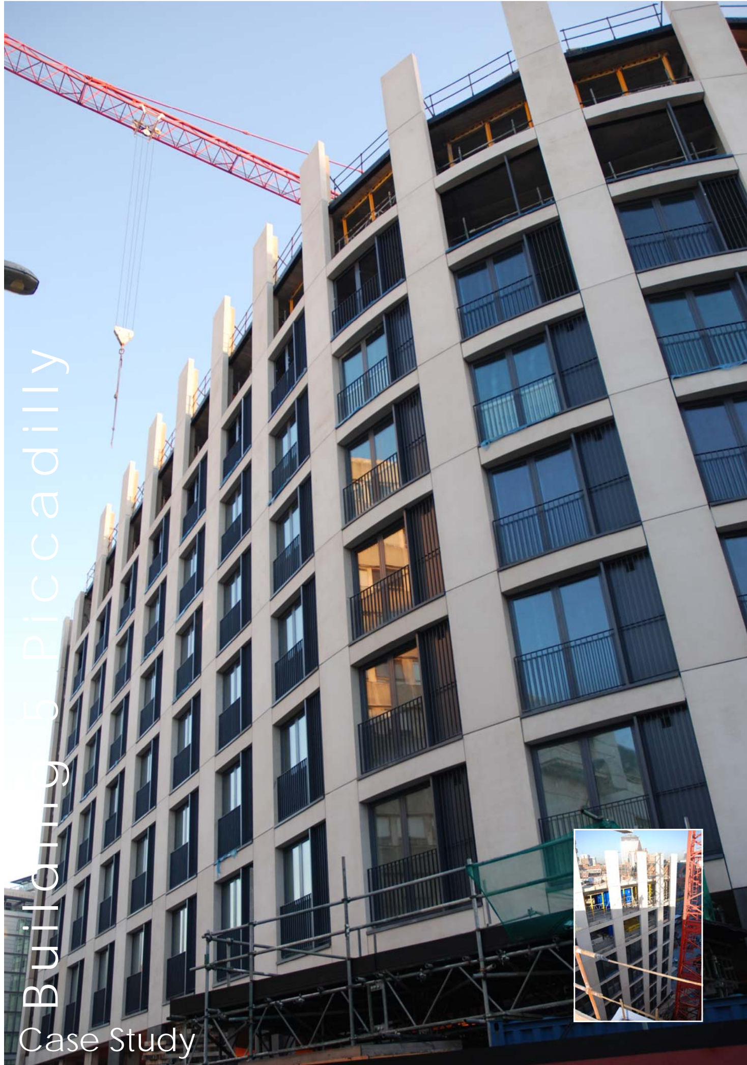
Structural cladding elements supplied as insulated sandwich panel.
