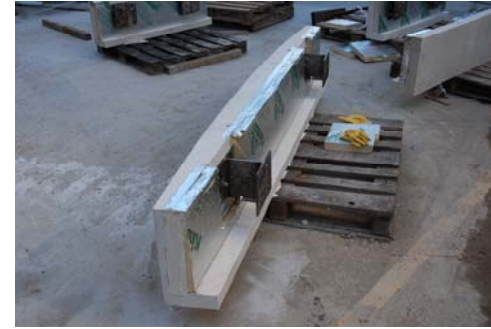
Spandrel panels are fixed back to edge channels with stainless steel bracketry.
