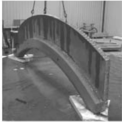
The segmental arch was designed as boot lintel to enable a 327mm faced soffit but keep the overall weight to a minimum.
