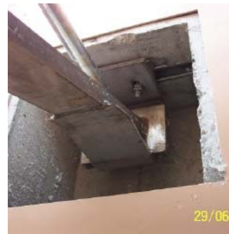
Stainless steel cast in channel securely held the units to the brackets.
