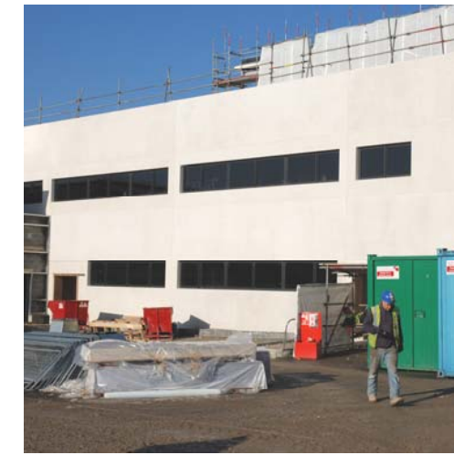
Typical cladding panels were 9 metres long and up to 4 metres high.
