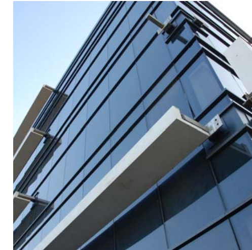
Projecting stainless steel bearers protrude through the curtain wall and are secret fixed in pockets at the end of units.
