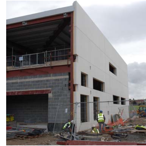
Steel frame detailed with fixing plates to provide lateral restraint to cladding panels.
