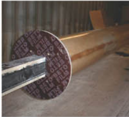
The frame was wrapped in flexible plywood, varnished and polished. From this, the fibreglass mould was layed up.
