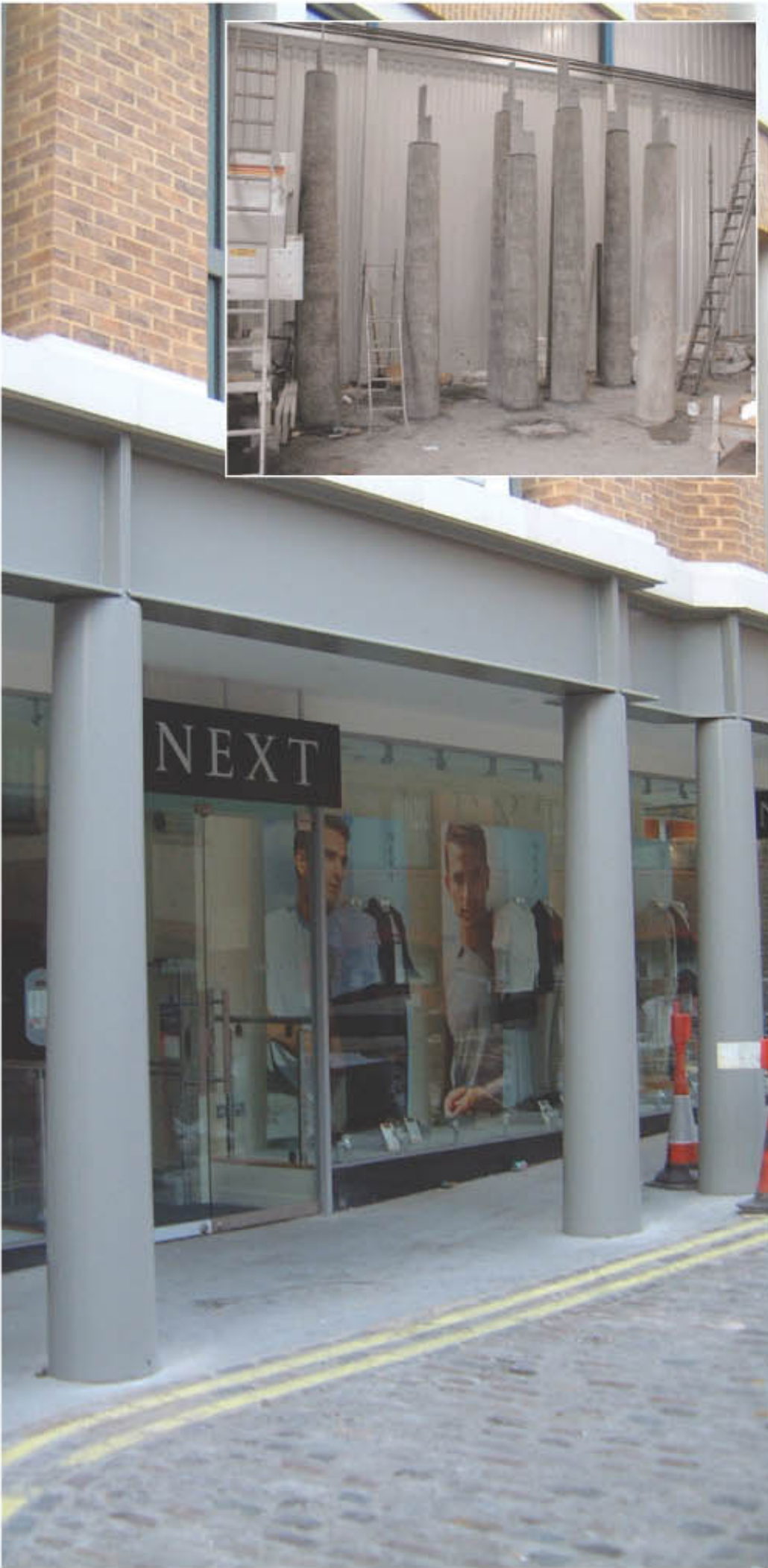
The plug for the fibreglass mould was made in-house using a steel core and decreasing timber loftings to create the taper.
