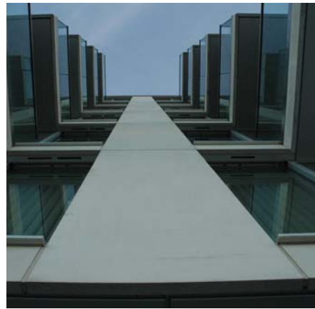
Vertically stacked mullion units manufactured as storey high cladding panels.
