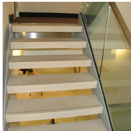
Internally individual step units were cast incorporating a stainless tread insert
