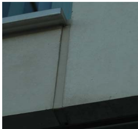
20mm mastic joint detailed with a 2mm recess. Non-staining Arbosil XL silicone sealant was specified.
