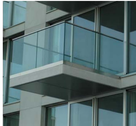
Projecting balconies manufactured from a steel frame cantilevered 2.4 metres and clad with spandrel panels.
