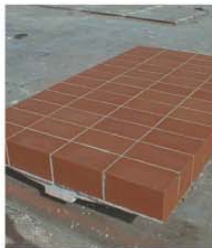
A typical canopy illustrating the terracotta corner return and stop end detail.
