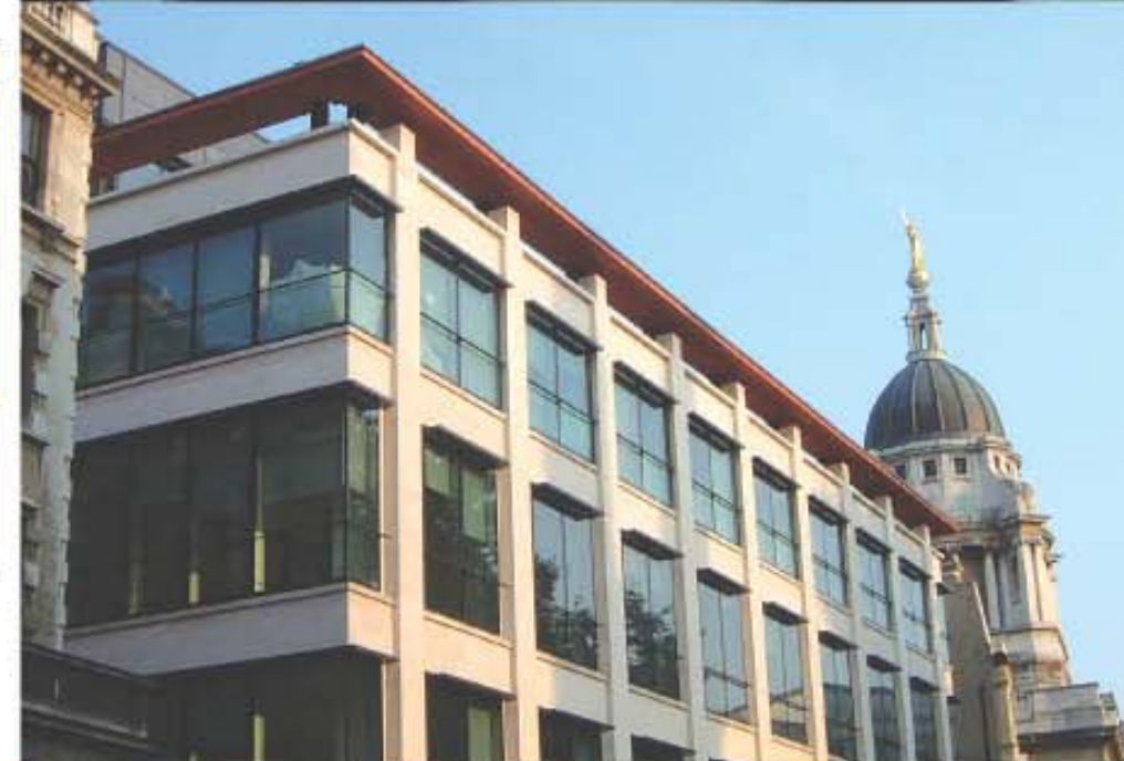
50% of all pieces supplied were corner returns. These were manufactured from standard tiles by water jet cutting mitres and fabricating back together with epoxy resin.
