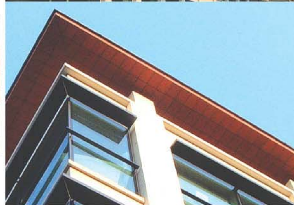
A typical canopy illustrating the terracotta corner return and stop end detail.
