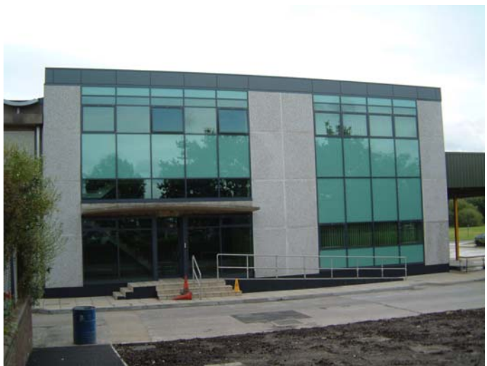
'Planar' glazing installed between precast elements provides the appearance of a contemporary new office development.
