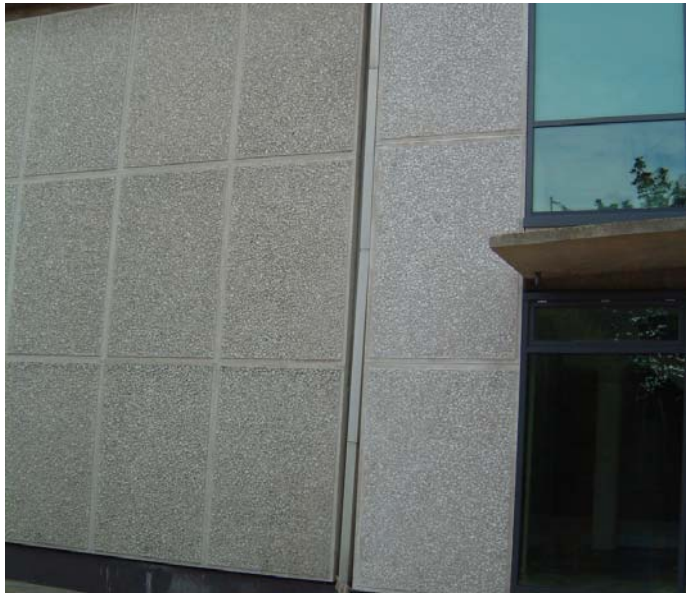
This photograph illustrates the match between existing cladding supplied in the 1960's and new panels supplied by Thorp Precast on the right.
