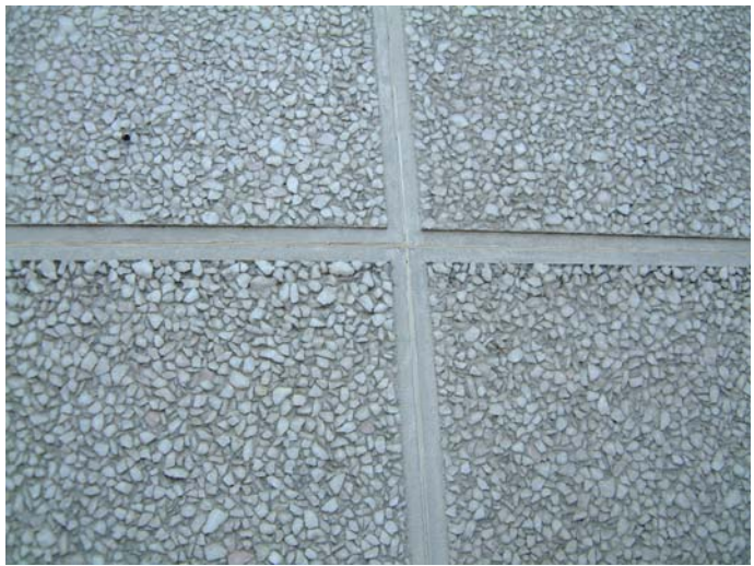
Panels are picture frames with a frame of fair faced concrete. 10mm joints were sealed with Arbosil XL silicone sealant. This specification ensures no discolouration of the white precast elements.
