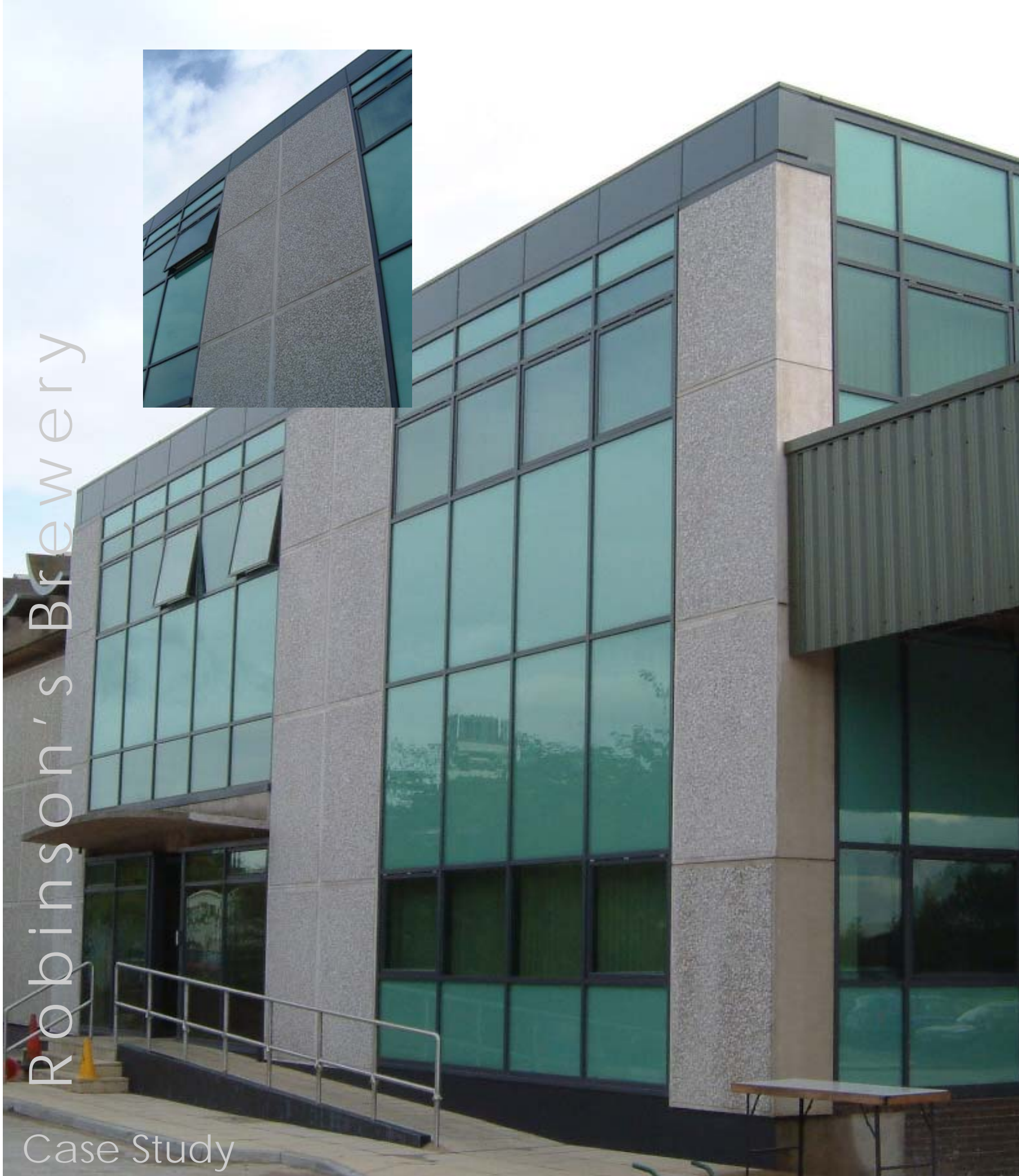
This photograph illustrates the match between existing cladding supplied in the 1960's and new panels supplied by Thorp Precast on the right.
